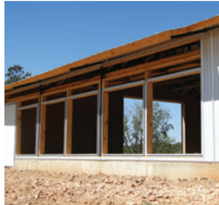
Fan framing is based on the number and size of fans for your project.
