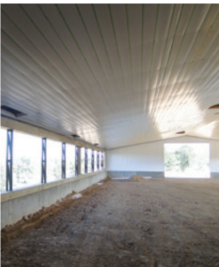
Tri-Ply material with blown cellulose or fiberglass insulation
