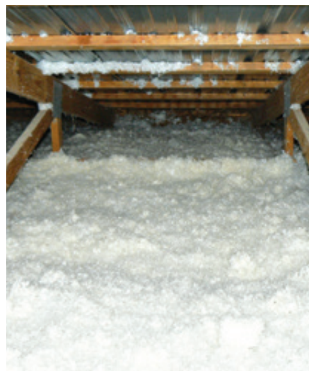
Blown fiberglass over Tri-Ply material in the attic of a drop ceiling house.
