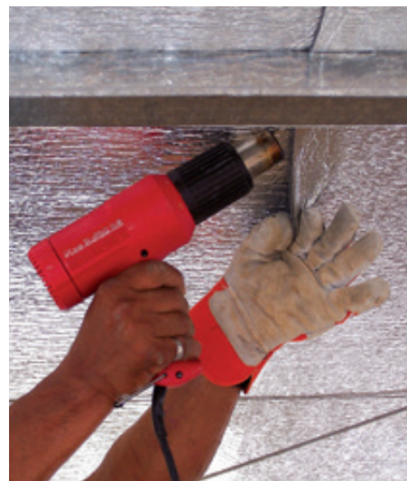
Reflective foil insulation material being installed as the drop ceiling.
